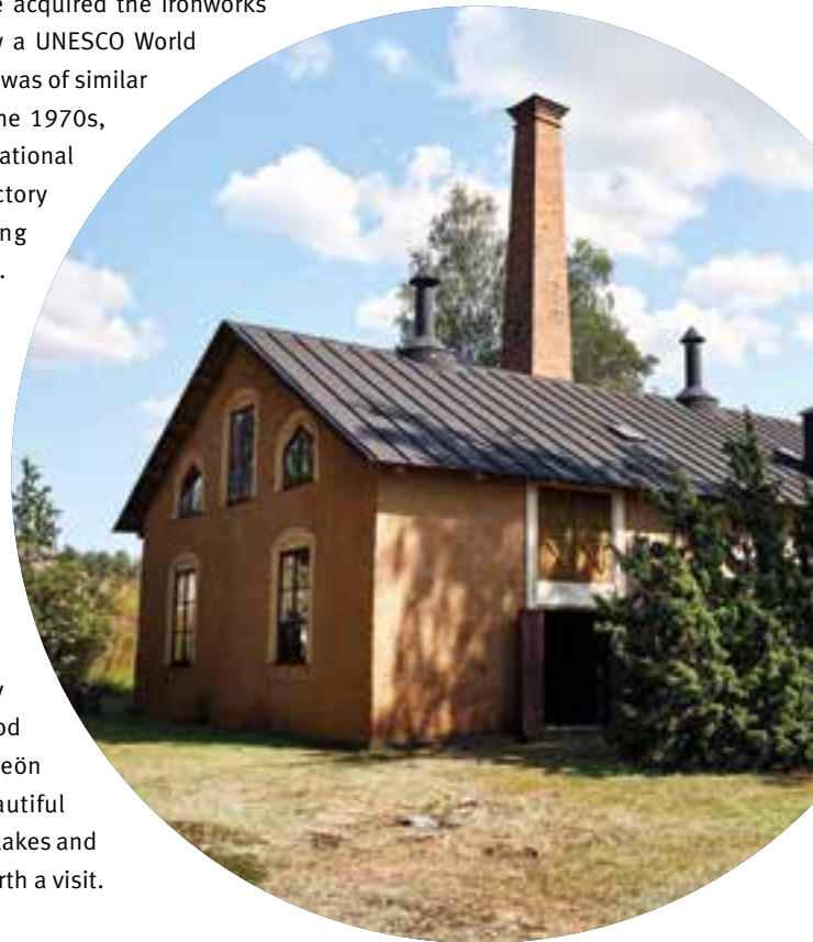
The old oil refinery at Oljeön island in Ångelsberg.
