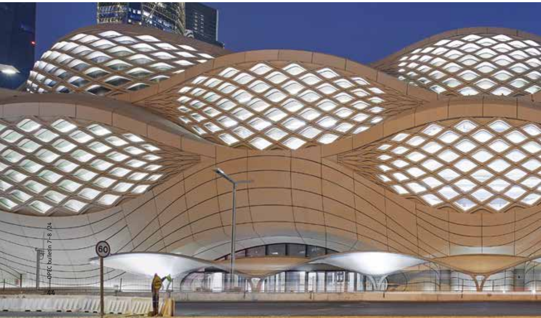
A rendering of the futuristic King Abdullah Financial District Metro Station in Riyadh.
