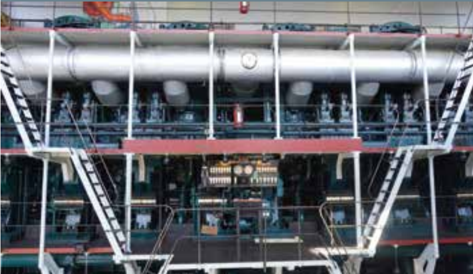
B&W 2000 is 24.6 meters long, 12.5 meters high and weighs 1,400 tons.
