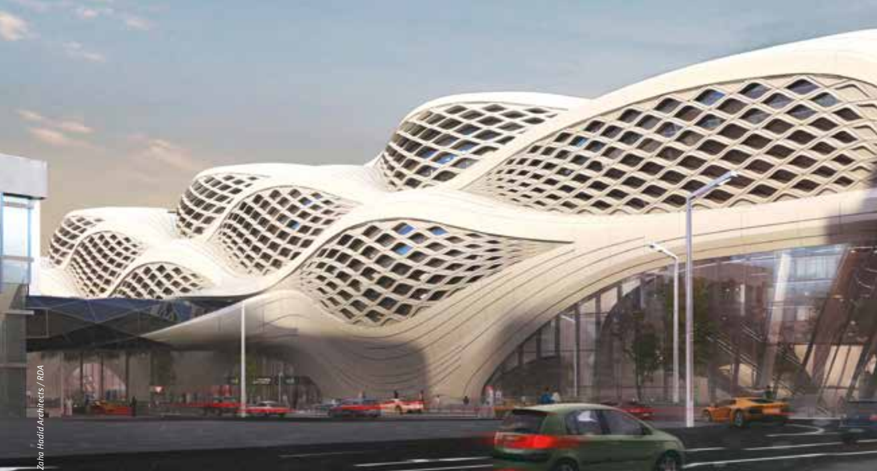
The Metro's ornate, latticed façade is designed to minimize sun exposure and optimize energy efficiency.
