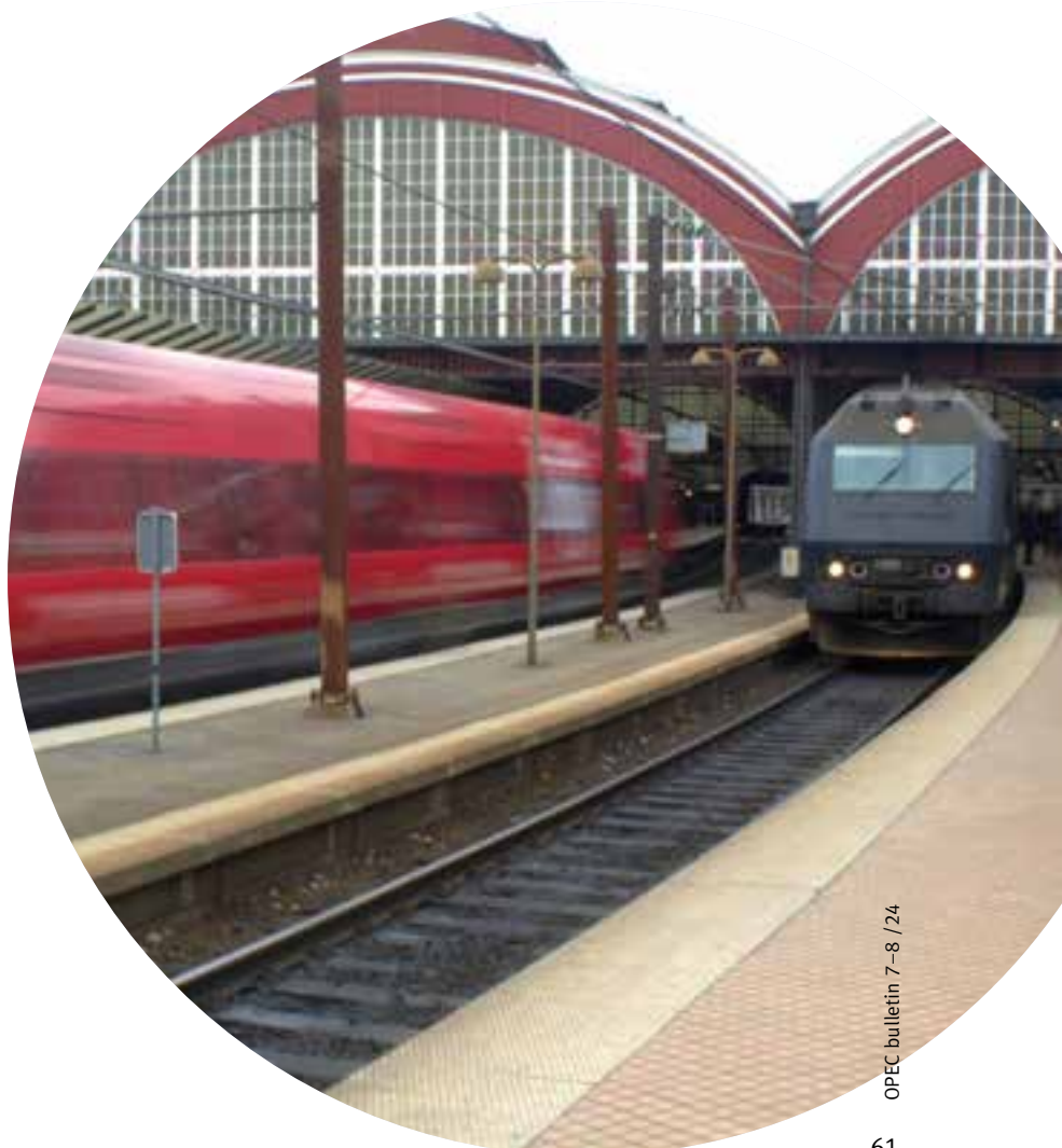
Railway station in Copenhagen.
