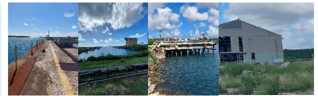
Figure 18 – Site visit photos
