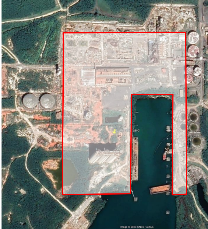
Figure 45 – Aerial photograph of the selected plot
